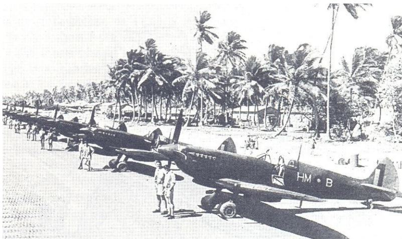
The well-know photograph of 'HM-B', variously identified as MT567 and MT657. (original source unknown.)
